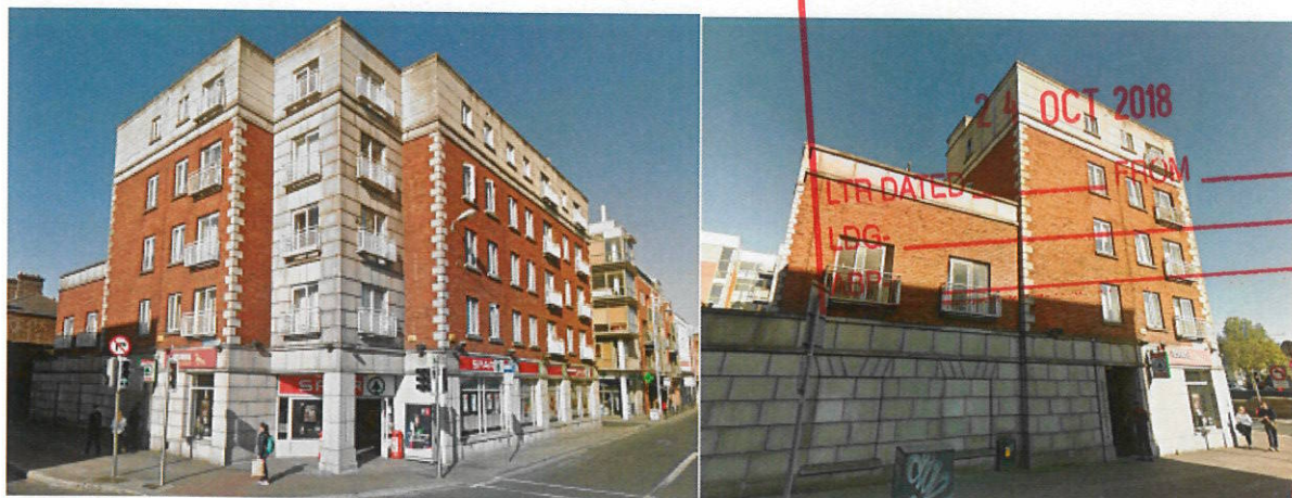
Figure 2.0 Image of the subject building at 'Chancery Hall' as viewed from Ellis Quay, Dublin 7.
